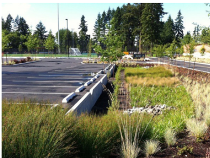
Vegetated Bioswales are Encouraged in Parking Lots
